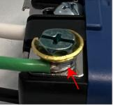
The ground wire wraps around the ground screw, under the brass washer. This is the only wire that wraps around a screw. The hot & neutral go into the wire holes and are clamped down as shown elsewhere on this page.
