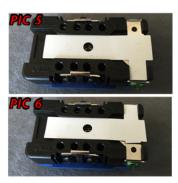
**Step 5.** Place trimmed gasket from Step 3 on back of outlet.
